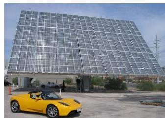
Figure 8: Amonix 7700 CPV system
