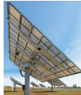
Figure 7: Concentrix Solar Flatcon CX-75 CPV system
